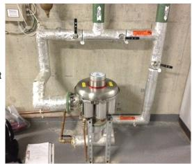
Below left is an EasyClean Automatic unit, built into a cabinet as part of a much larger system including UV disinfection for toilet flushing.
