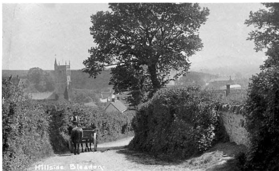
Hillside - top of Celtic Way
