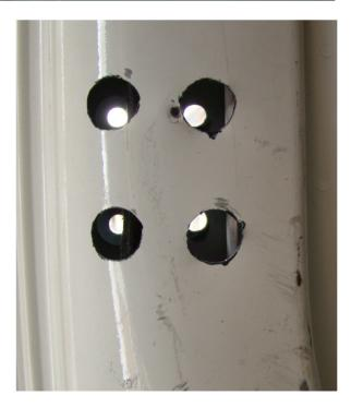
Place washers on socket screws, then pass the socket screw through the top left hole and screw into moal lock. Place the bottom left socket screw through and tighten, leaving some play in movement. Then place a sliding nut (raised side facing inwards) through the moal lock and put a socket screw through it. Repeat this for last bolt. Tighten all bolts, this side of the moal lock is now fitted.
