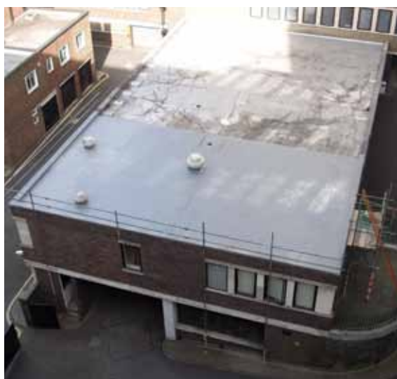
Watertight: a recently-completed project at Grosvenor Place, using Cap Roofseal
