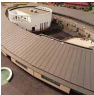
Front cover: Middleton School, Milton Keynes is an exemplar of modern school construction under the Building Schools for the Future (BSF) programme. The multi-geometry roofs comprise 30-year durability single ply membrane on high-performance insulation supported by a profiled metal deck. The job was completed by SPRA member Voland Roofing with Leadbitter Construction as main contractor. (Photo courtesy of SPRA)
