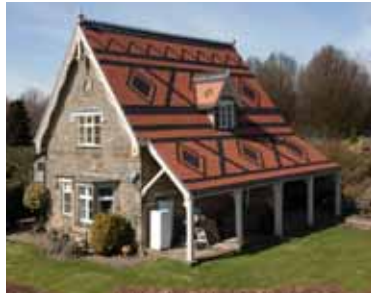
Front cover: Swiss Cottage at Castle Howard, where Dodds Roofing Services Limited fitted Sandtoft Humber clay plain tiles in a diamond formation using spearhead tiles and finial ridges in two colours.
