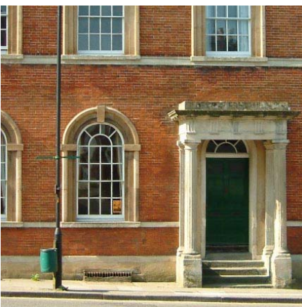
High quality brickwork, often with stone dressings, is a particular feature of many Georgian and later buildings in Devizes. The window surrounds here in Long Street are cast imitation stone.
