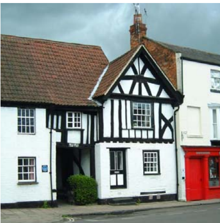
Although Great Porch House dates from the 15 th century many of the external features such as the Georgian sash windows are later.
