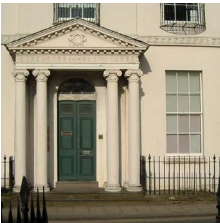
The refinement of the late 18 th century with slim glazing bars to the sash windows and contemporary wrought iron railings. Ionic columns support the elaborately detailed pediment to the front portico. The finish is painted stucco.
