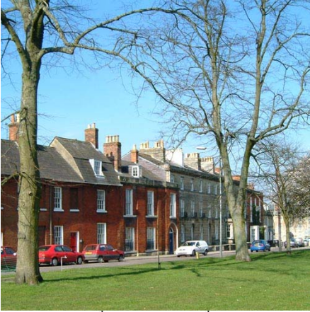
These late 18 th and early 19 th century brick and stone houses at Southbroom Terrace enjoy an open aspect over The Green.
