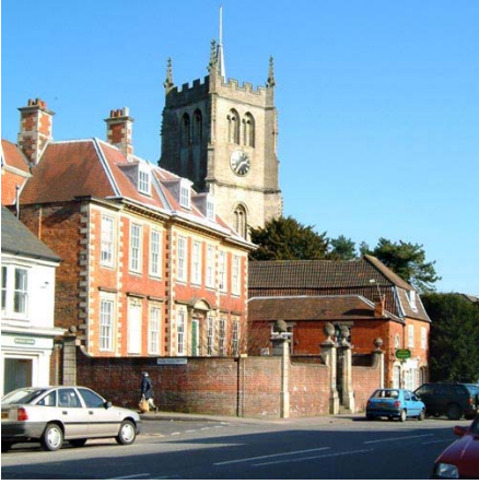
Brownston House is one of the high status buildings of Devizes and is typical of the style and materials used in the 18 th century. Gates and gatepiers complement the setting.
