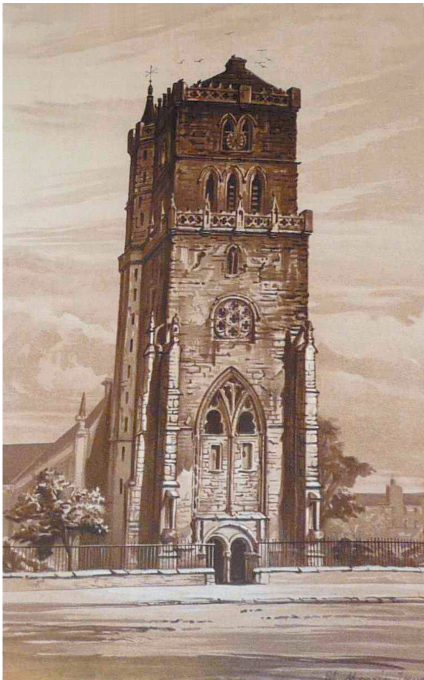
Steeple before the 1870 restoration, taken from the west and showing the entry doors to the Steeple Church and tower.
